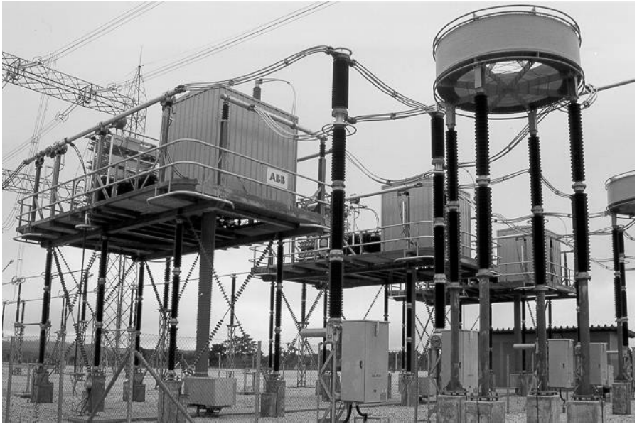
Fig. 1.19. TCSC (Source: ABB)
