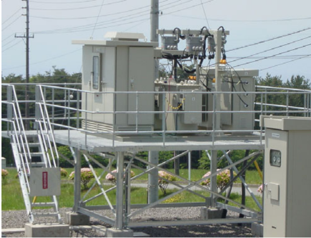
Fig. 16.14. Installation of a 6.6 kV – 100 kVA BTB type LPC for DAPS simulator
